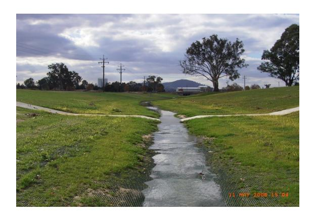
TRM's capture sedimentation and filter water flows through natural vegetation for cleaner waterways.
